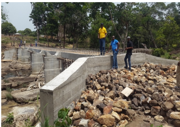
Construction of Kundi Bridge, kono District
